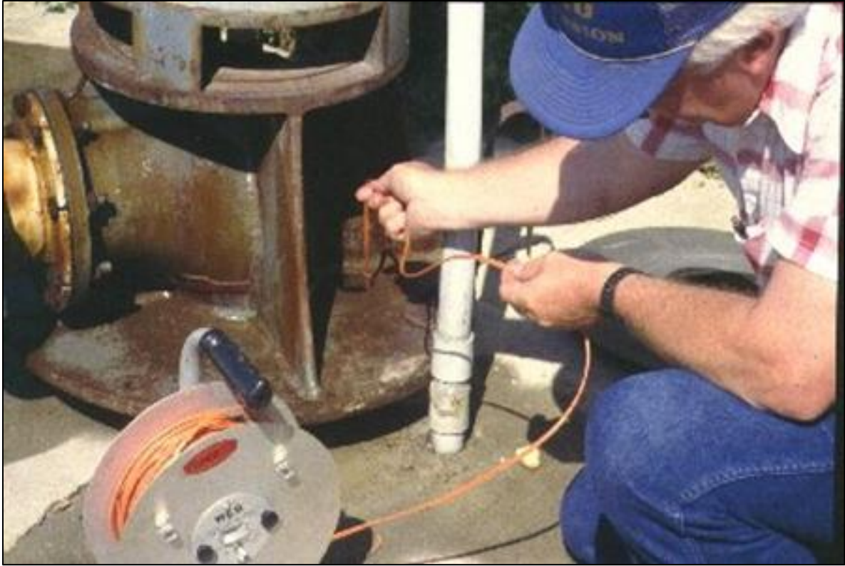
Figure 4.3 - Well access hole for measuring water levels.
