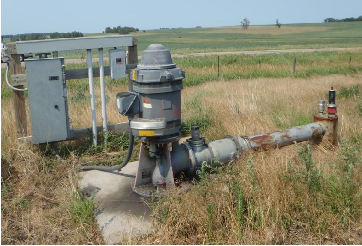
Figure 3.13 - Vertical hollow shaft electric motor driving a vertical turbine pump.
