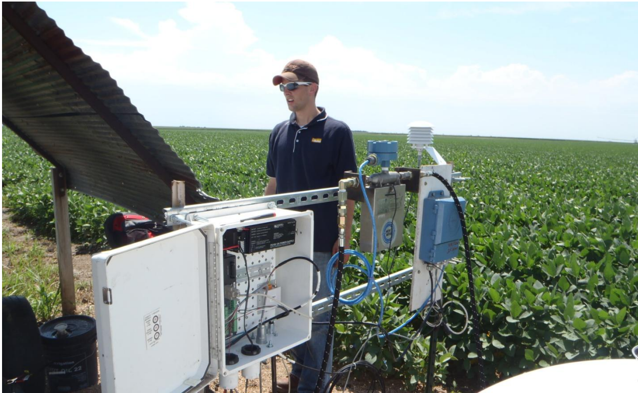
Figure 4.12 – Coriolis flow meter used for pumping plant test.
