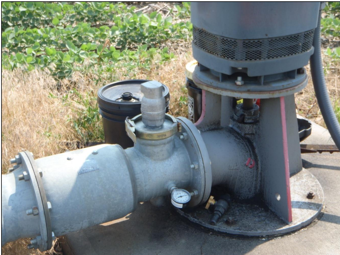
Figure 4.6 - Pressure gauge installation on well discharge pipe.
