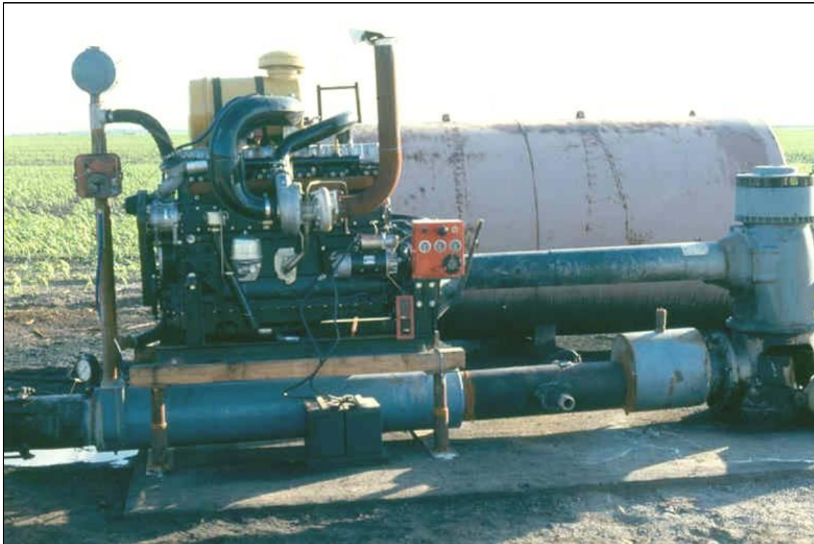
Figure 3.3 - Diesel powered turbine pump with right angle drive.
